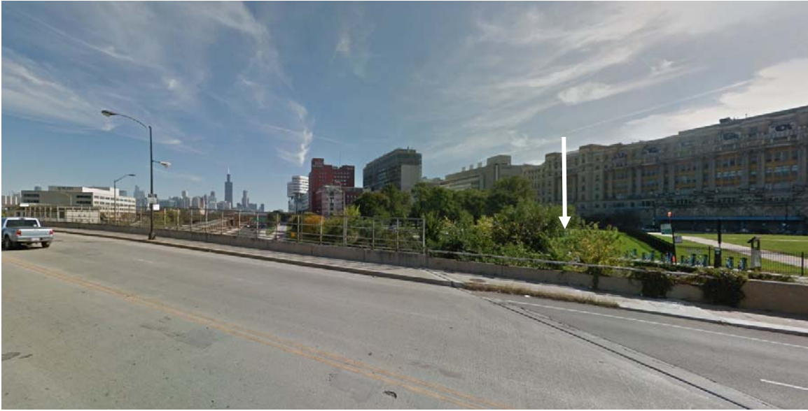
View east along West Ogden Avenue bridge and I-290 Preferred Alternative (at left), B83 noise barrier location (arrow location at right), and north-facing facade (at right).
