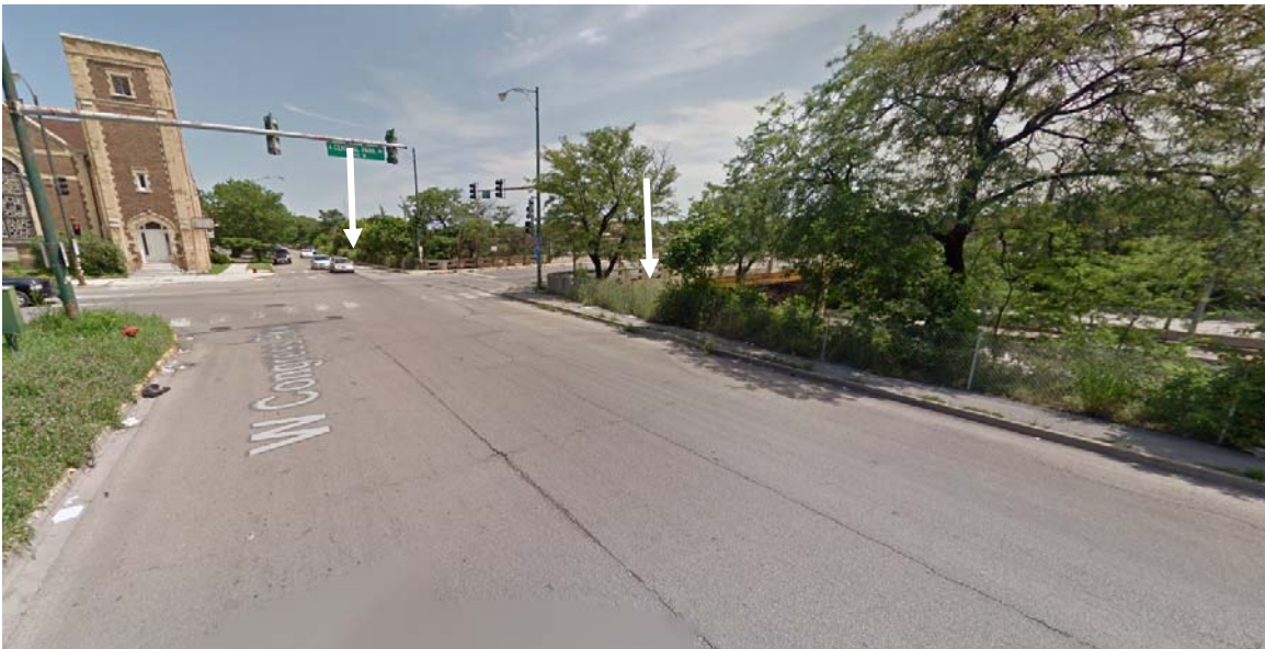
Figure 4-56. First Church of the Brethren
