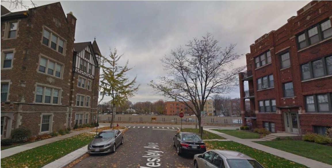
View north along Wesley Avenue toward Garfield Street, I-290 Preferred Alternative (at center), and east-facing facade (at left).
