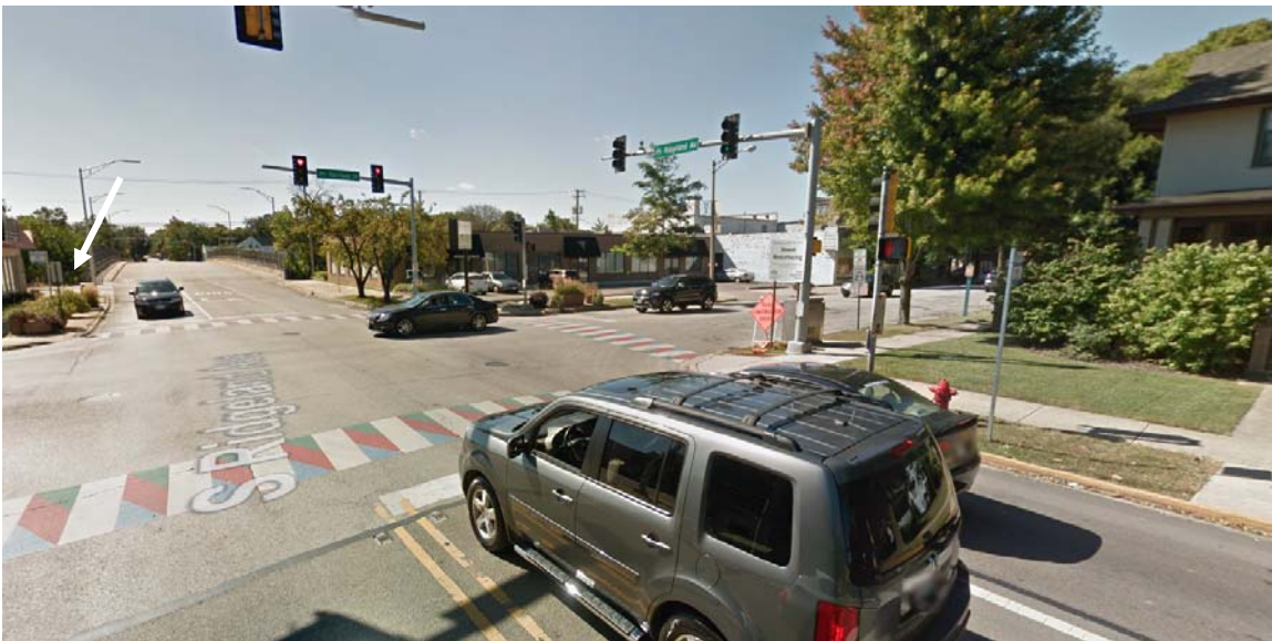
View southwest along South Ridgeland Avenue at Harrison Street from district's east NRHP boundary toward contributing building on South Ridgeland Avenue (at right), I-290 Preferred Alternative (at center), and South Ridgeland Avenue bridge (at center). B38 noise barrier location (arrow location, at center) along I-290 north right-of-way, east of South Ridgeland Avenue bridge.
