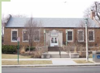
Maze Branch Library 845 S. Gunderson Ave., Oak Park Criteria A, B, C
