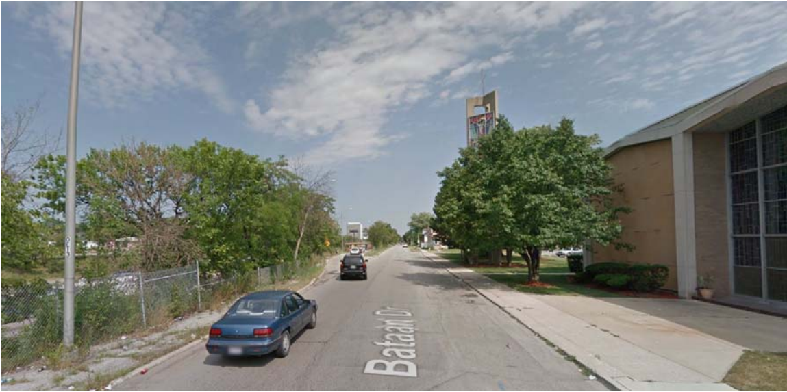
View east along Bataan Drive (frontage road) to I-290 Preferred Alternative (at left), B17 noise barrier location (at left, center along existing fence), entrance ramp (at center), and north-facing facade (at right) from South 9 th Avenue.
