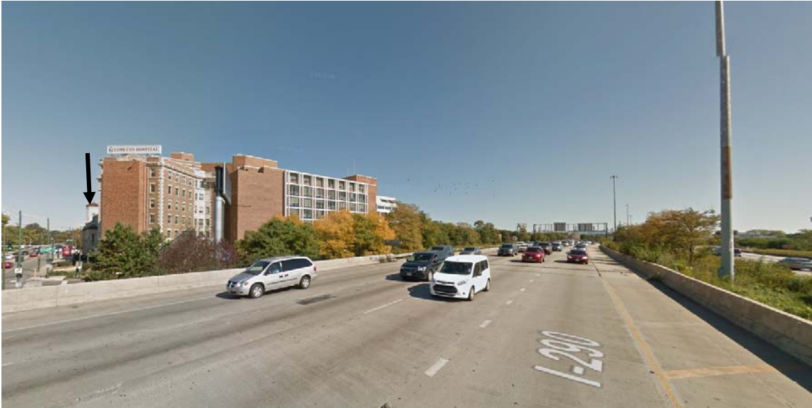
View northeast along I-290 Preferred Alternative westbound travel lanes, east of South Central Avenue, toward Loretto Hospital (at left, center) and Assumption Greek Orthodox Church (arrow location, at left). B44 noise barrier location (at right) within I-290 right-of-way, in median between eastbound and westbound travel lanes.
