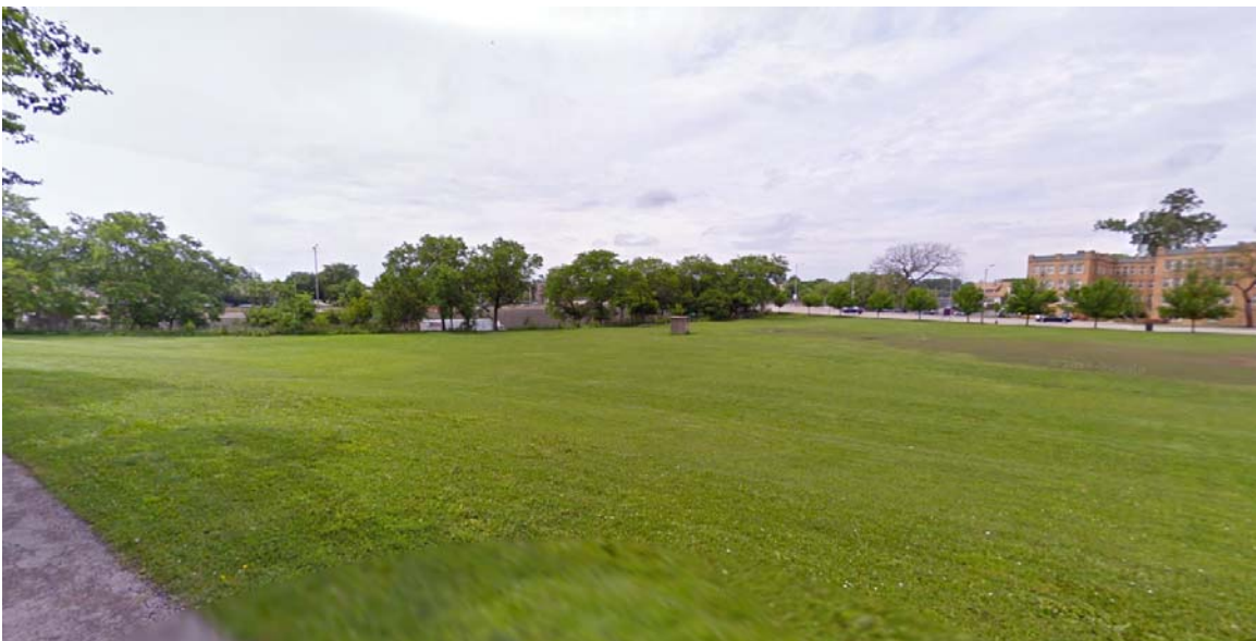
View southwest along existing park trail from within Columbus Park toward its southwest corner and proposed shared-use path connection (center), South Austin Boulevard (at right), I-290 Preferred Alternative (at center), and B40 noise barrier location west of South Austin Boulevard.
