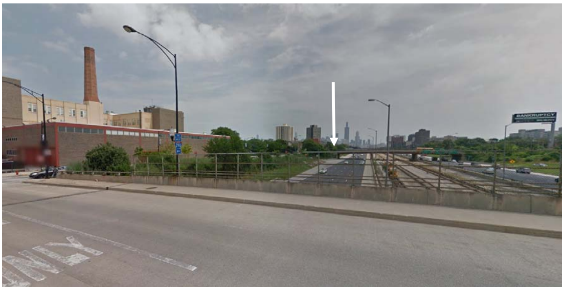
Figure 4-68. Crane Technical High School
