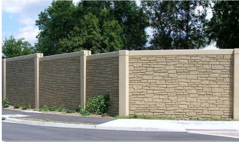
Figure 4-1. IDOT Frequently Used Wall Type
