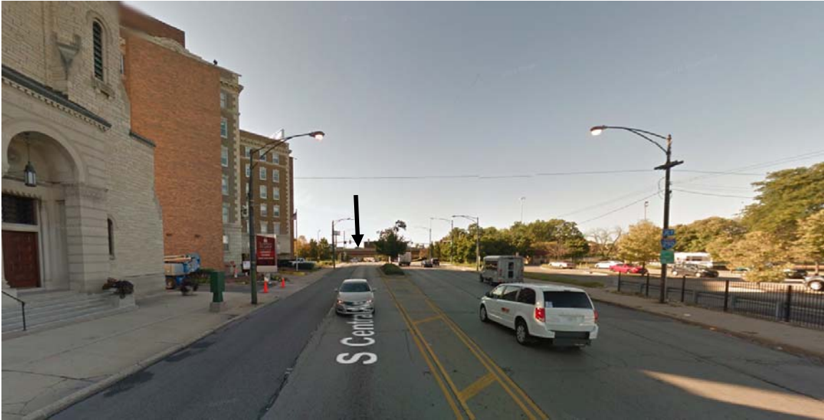
View south along South Central Avenue from west-facing facade (at left) toward I-290 Preferred Alternative (at center), South Central Avenue bridge (arrow location, at center), and Columbus Park (at right). B44 noise barrier location (left of arrow location, east of South Central Avenue) within I-290 right-of-way, in median between eastbound and westbound travel lanes.
