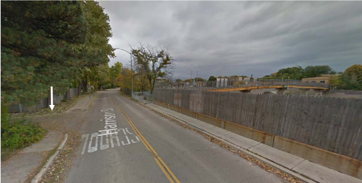
View southeast along Harrison Street toward I-290 Preferred Alternative (at right), pedestrian bridge (at right, center), and district's southwest NRHP boundary along alley between Clinton and Home Avenues (arrow location, at left). B31 noise barrier location at right, along existing fence at I-290 north right-of-way and west of pedestrian bridge.
