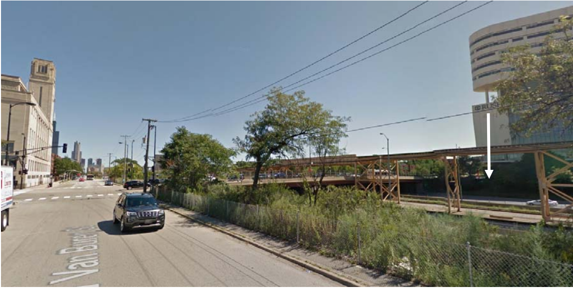
View southeast along West Van Buren Street toward South Ashland Avenue, (at center), I-290 Preferred Alternative (at right), and west-facing facade and south side elevation (at left). B83 noise barrier location along south I-290 right-of-way, west of South Ashland Avenue (arrow location at right).
