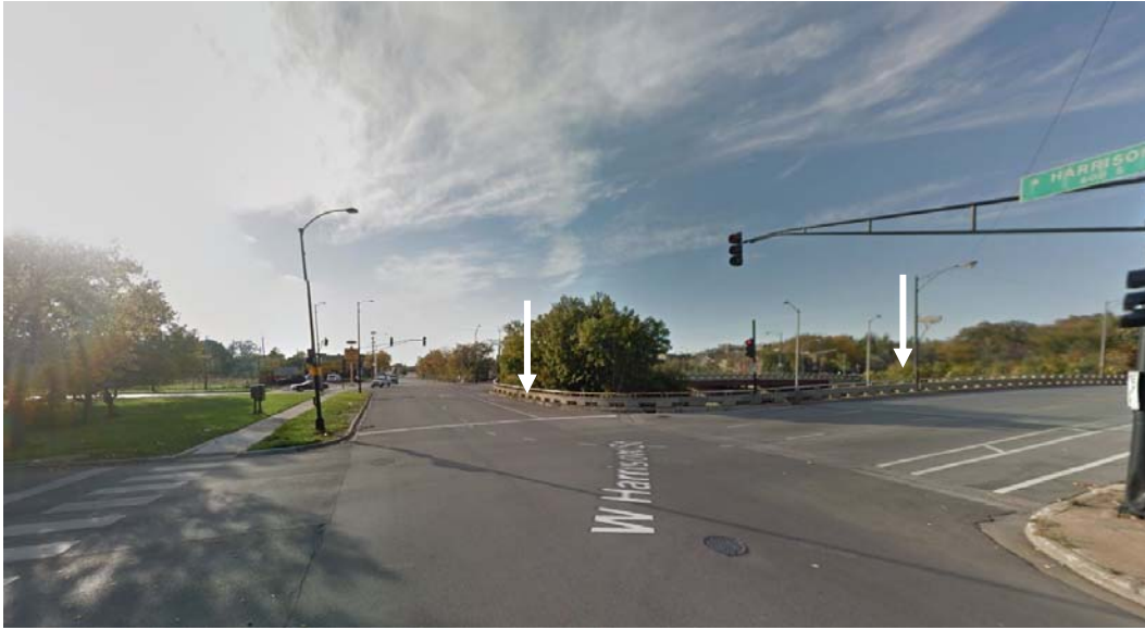
View northwest along West Harrison Street at South Independence Boulevard (at center) within Chicago Park Boulevard System Historic District boundaries toward I-290 Preferred Alternative (at left). Noise barriers along I-290 north and south right-of-way (arrow locations).
